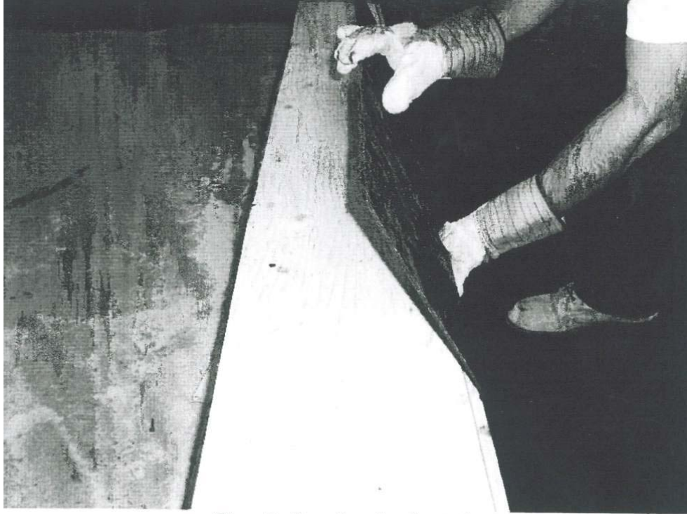
Step 3: Bending the board.
