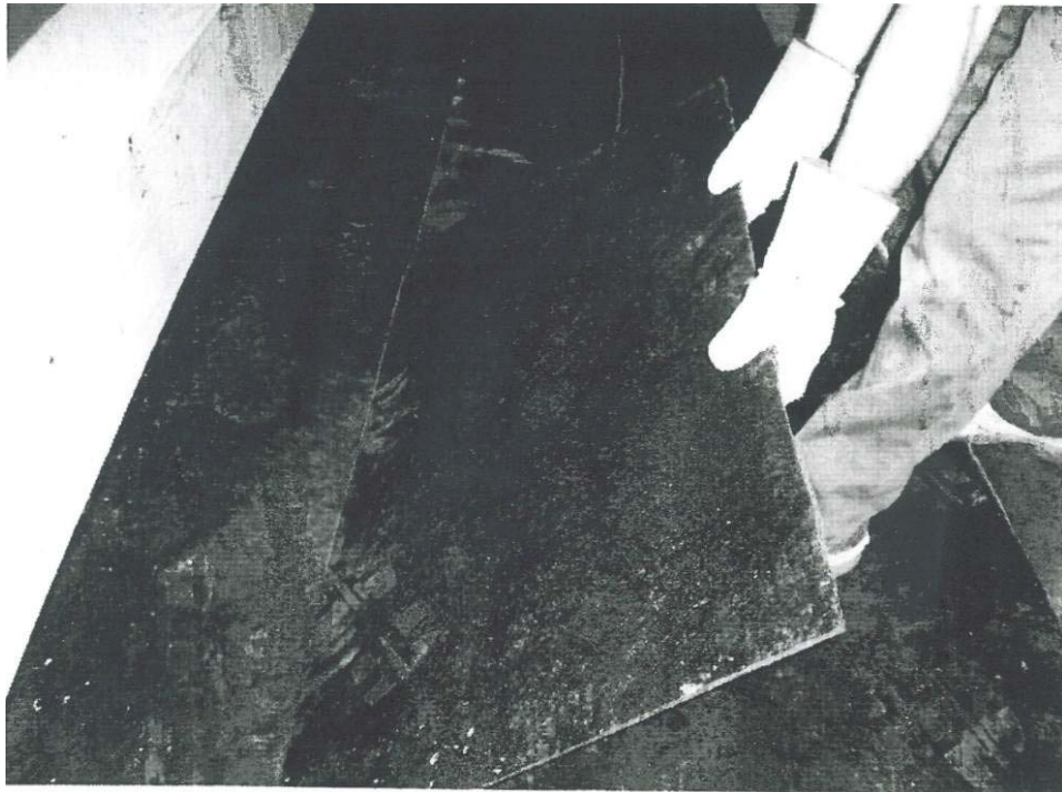
Step 2: Installation on the parapet.
